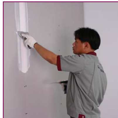
6. Cover the screw head and joint with Easy Joint Compound.
