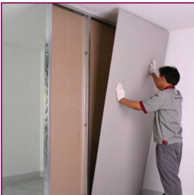
5. Screw Gypsum Board to the frame leaving 10 - 16 mm. space from board edge. Each screw will be 20 cm. apart. In the middle of the board, each screw will be 30 cm. apart. Use black screw 25 mm. for a single layer partition and 38 mm. for double layer partition. Second sheet and joints of both layers need to be staggered.
