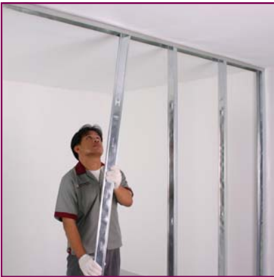
3. Attach C75 into U76 at every 60 cm. space
