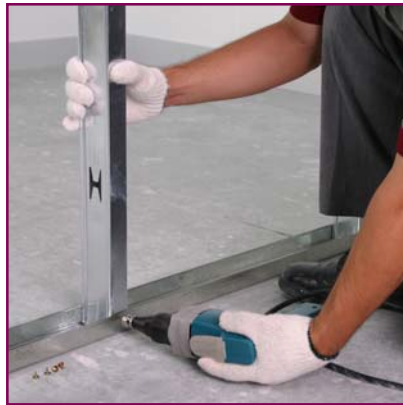
4. Attach the end of C75 to U stud by using reweigh or screw
